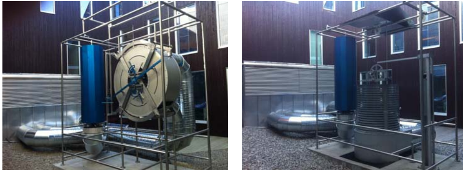
Figure 2A and 2B: 2A: Step two 'Pulse' real-size installation on site; first version. It was a failure because the air from the ventilation system did not move the hammer. Figure 2B: Step three: 'Pulse' real-size installation on site; second version, including a frictionless bellows, and where all functions were safeguarded and resolved according to the original concept
